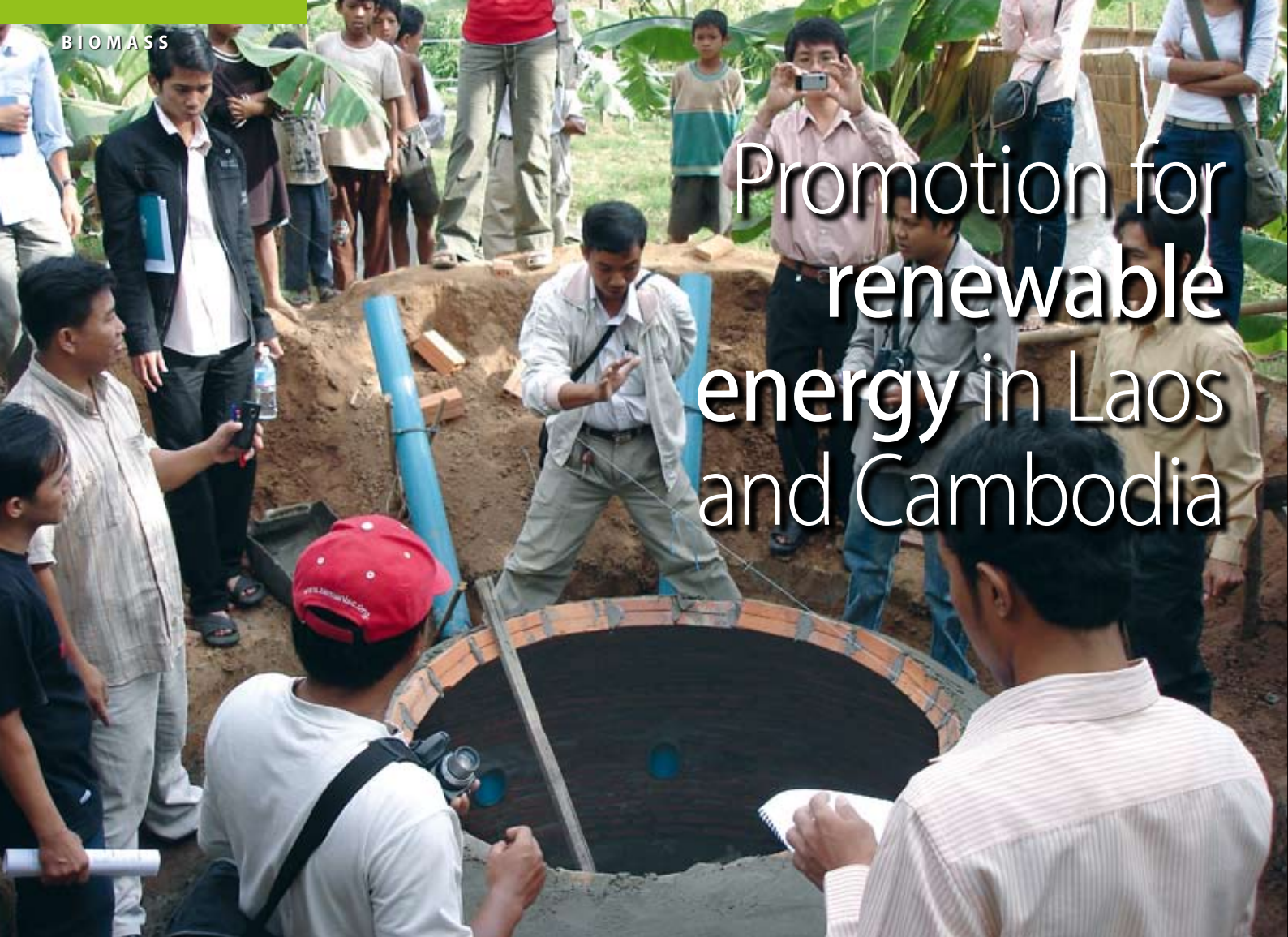
Construction of a 4 m 3 biogas plant in Cambodia
