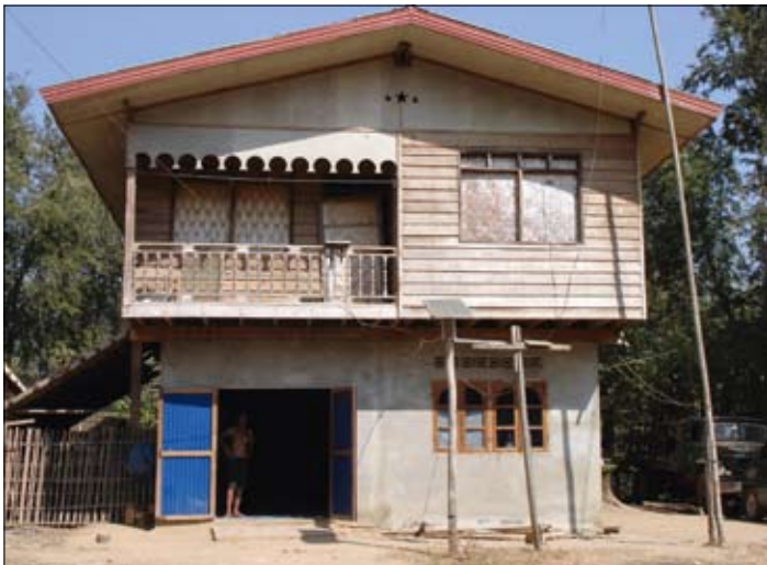
Common solar home system in Laos
