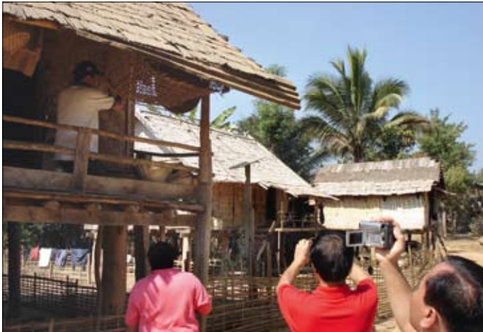
This solar home system in Laos is shadowed.
